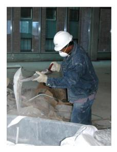
When debris from the demolition is dropped through holes in the floor without the use of chutes, the area where the material is dropped must be enclosed with barricades at least 42 inches high and at least 6 feet back from the projected edges of the opening above.
